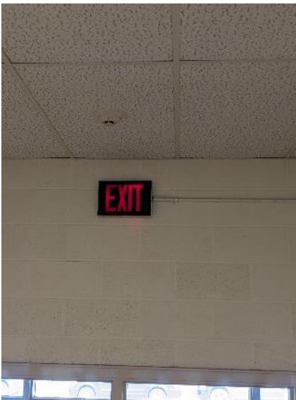
Examples of exit signs and emergency lights that require annual testing.
