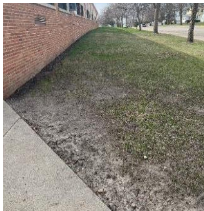
West side of building.
