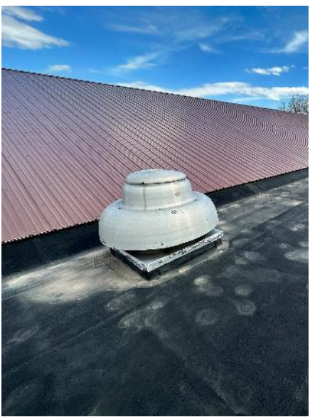
Power Roof Ventilators
