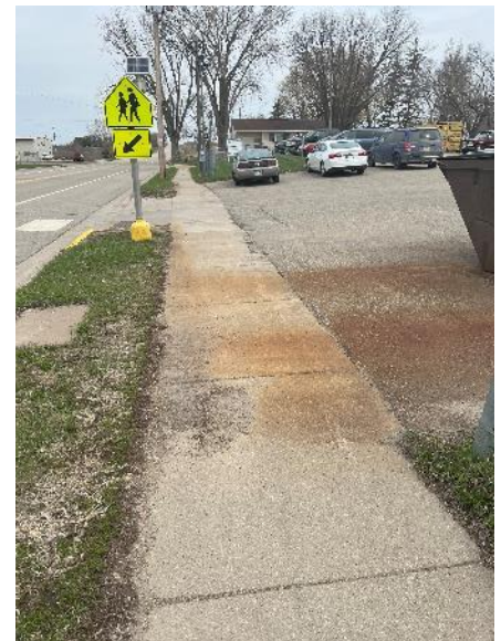
Shared pedestrian crossing and parking lot entrance.
