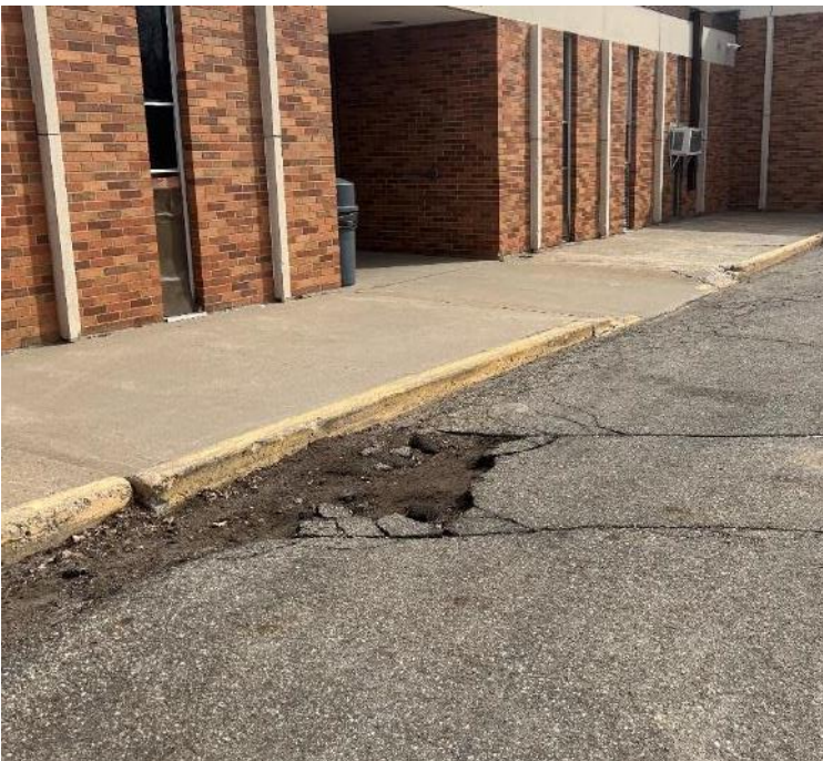
Curb in front of the south facility entrance.
