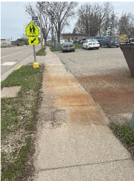
Parking lot entrance along CSAH 1.
