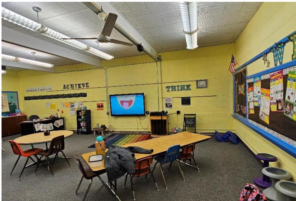
*Standard classroom with lack of white boards, dated technology, limited access to power, and non-flexible furniture
