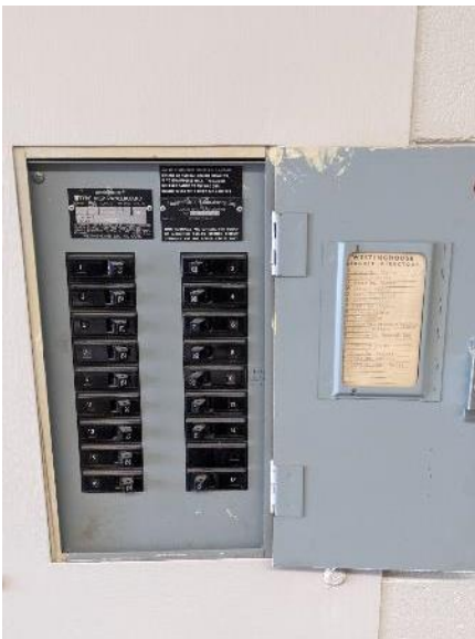
Panel in Corridor 101 outside Music Rm 159
