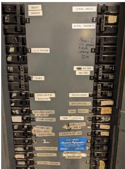
Examples of panels needing updated labels and circuit directories
