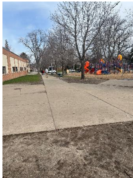
Storm sewer to outlet to the north.
