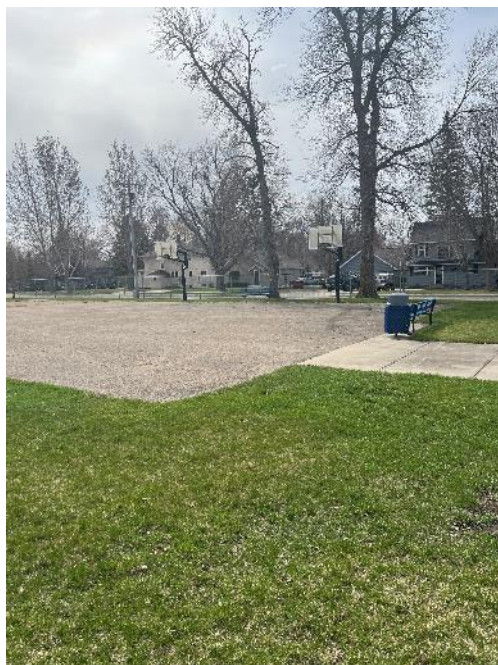
Basketball court bituminous pavement.
