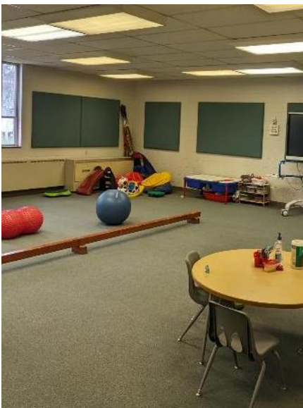
ECCE – Unit Ventilators
