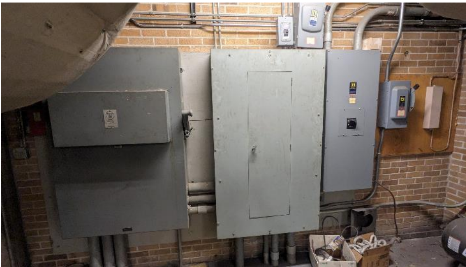
240V, 3-phase Service Disconnect (Far Left) and Distribution Panel (Center) – Both are Westinghouse branded equipment and should be replaced.
