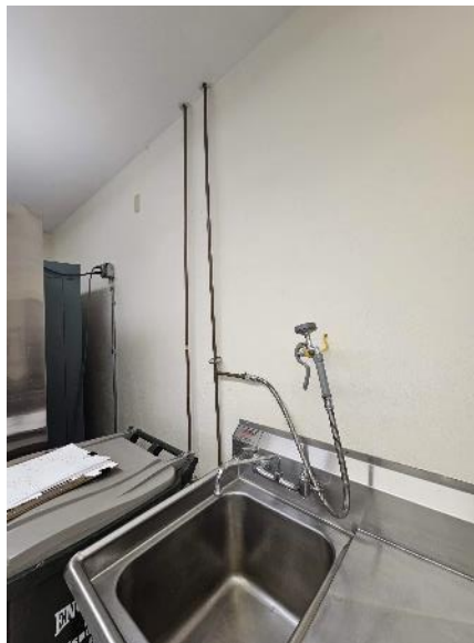
Reroute and insulate water lines.
