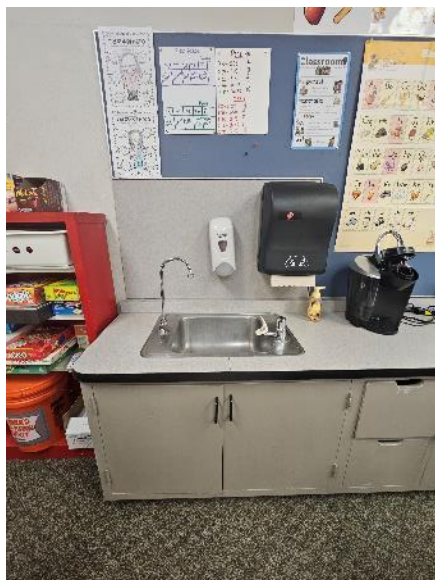
Non-accessible sinks & surface heights
