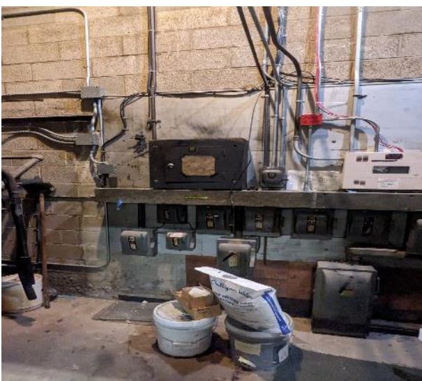
Square D Panel and Equipment Disconnects in Furnace Room 119.
