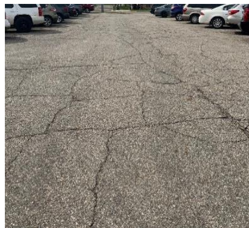
South parking lot looking south.
