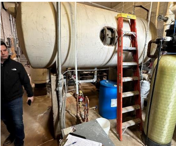
Shell and Tube Heat Exchanger
