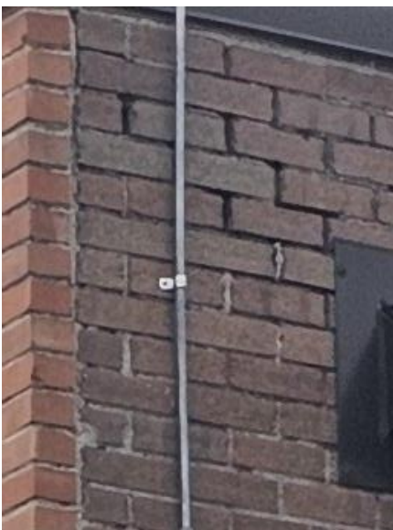
Joint / Tuckpoint repair
