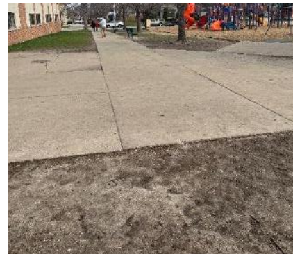
Courtyard area looking north.
