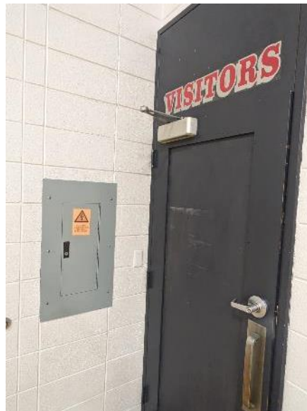
Panel B in North Wall of Gymnasium 14E
