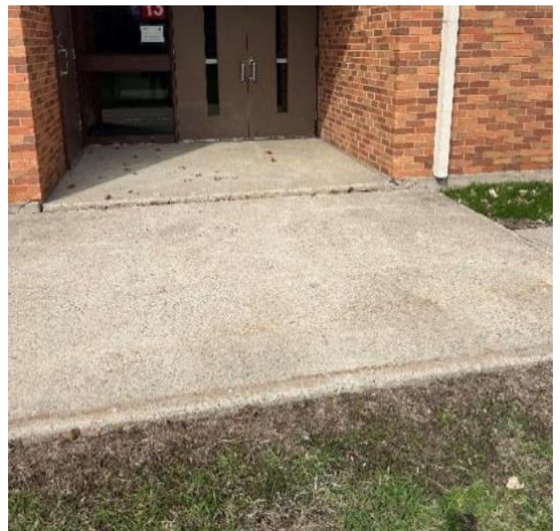
East building entrance (door 13).
