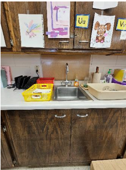
Non-accessible sinks & surface heights
