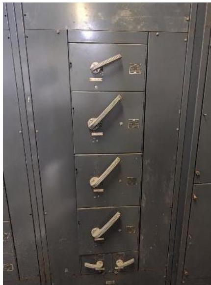
Existing 2000A ITE Switchboard for Electrical Service Entrance
