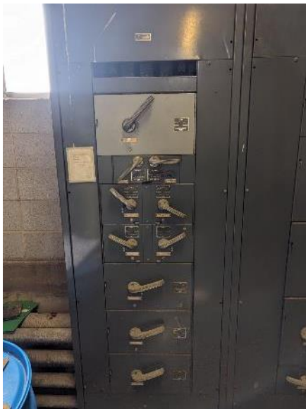
Existing 2000A ITE Switchboard for Electrical Service Entrance
