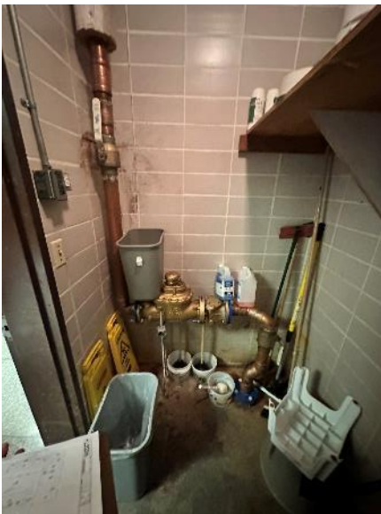
Replaced water service
