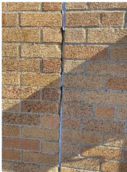
Deteriorated joints
