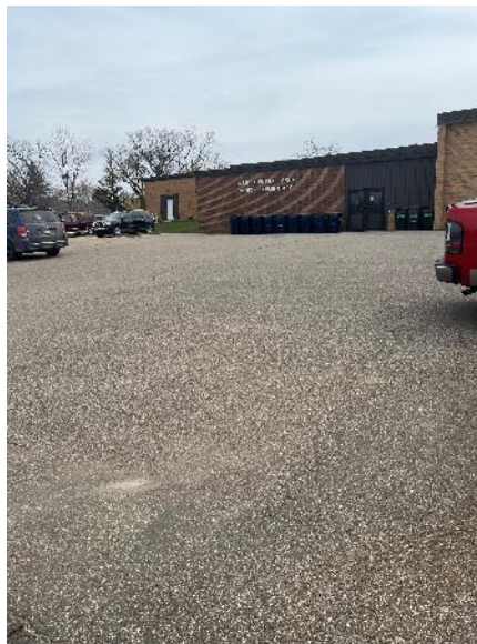
Parking lot on the west side of the facility.
