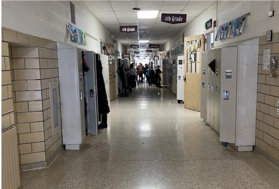
*Double loaded corridors, with lockers and poor sightlines and security.
