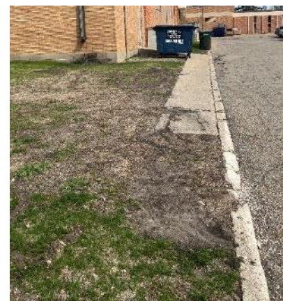
South side of facility.
