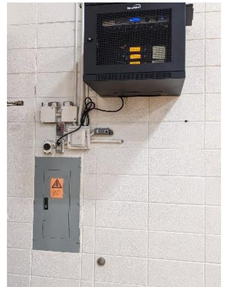
Panel C in South Wall of Gymnasium 14E
