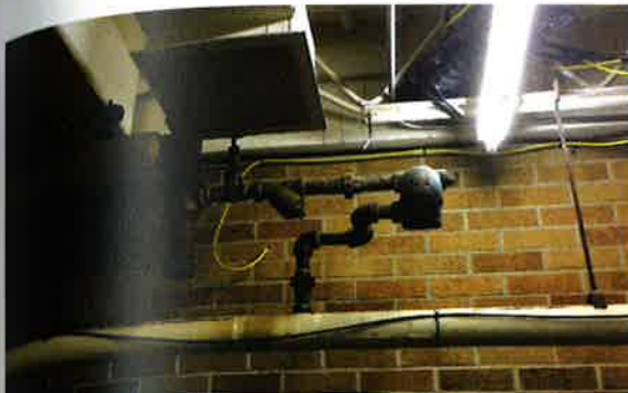
Old steam heating coils, steam traps, and piping will be removed...
